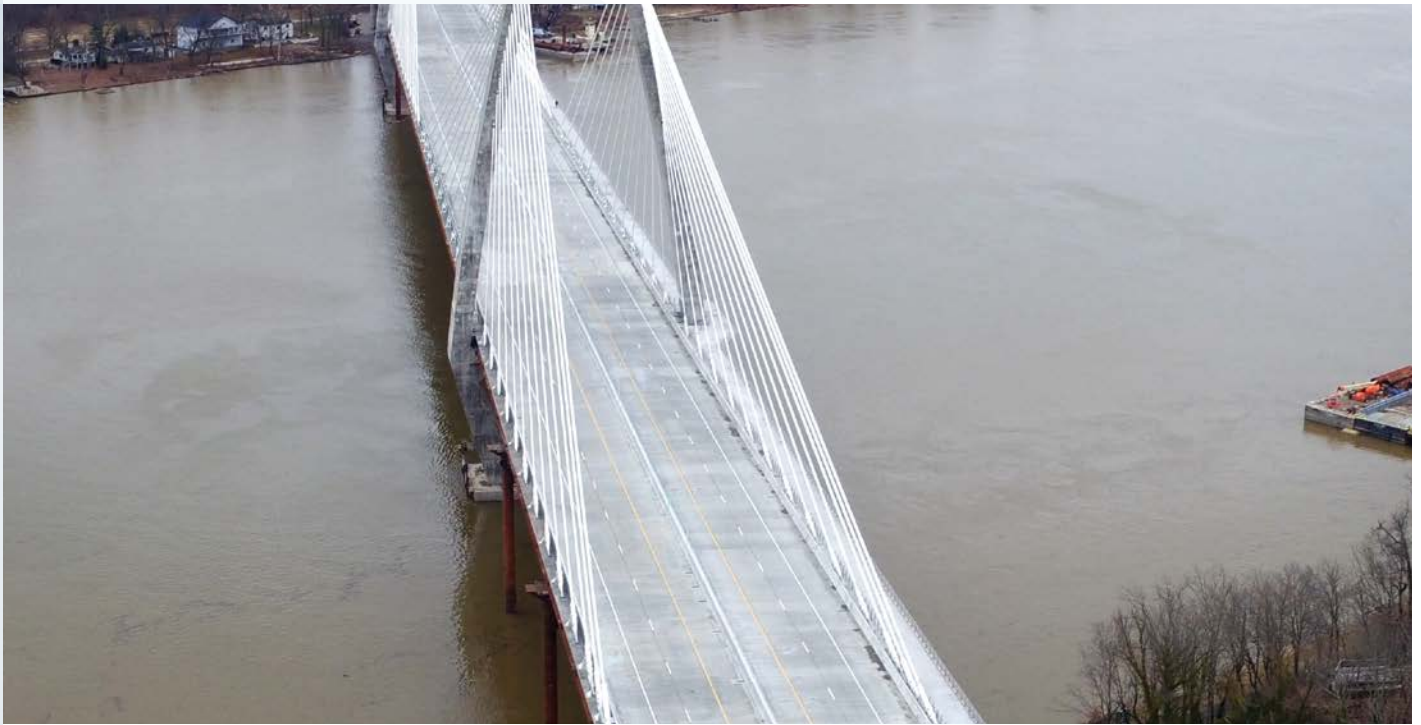
Ohio River Bridge, United States of America
