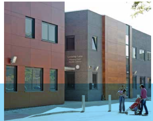
Clockwise from top: Gloucester Hospital, UK; Primary Health Care facilities, Barnet, Enfield, UK; Marrngoneet Correctional Centre, near Melbourne, Australia.
