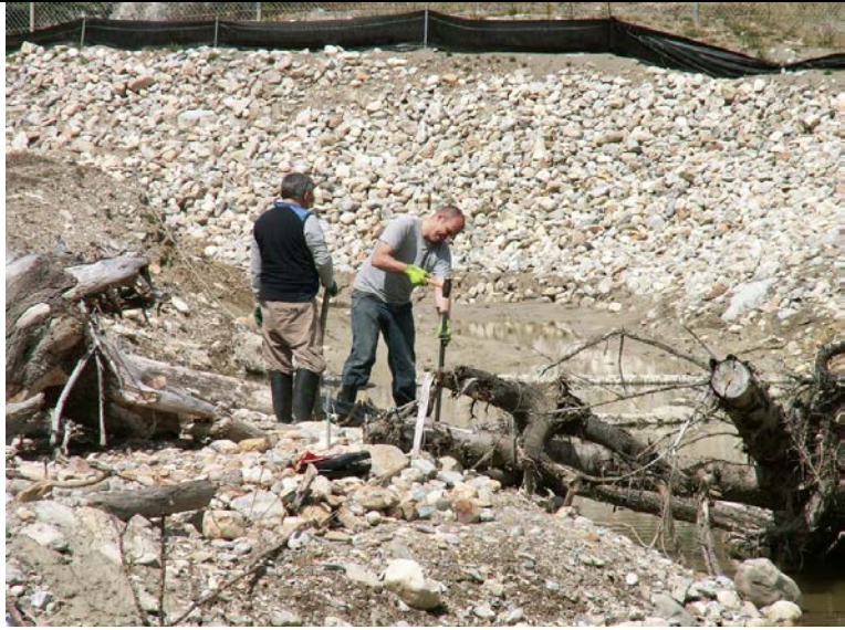
Volunteers digging holes for willow staking at constructed pond.
