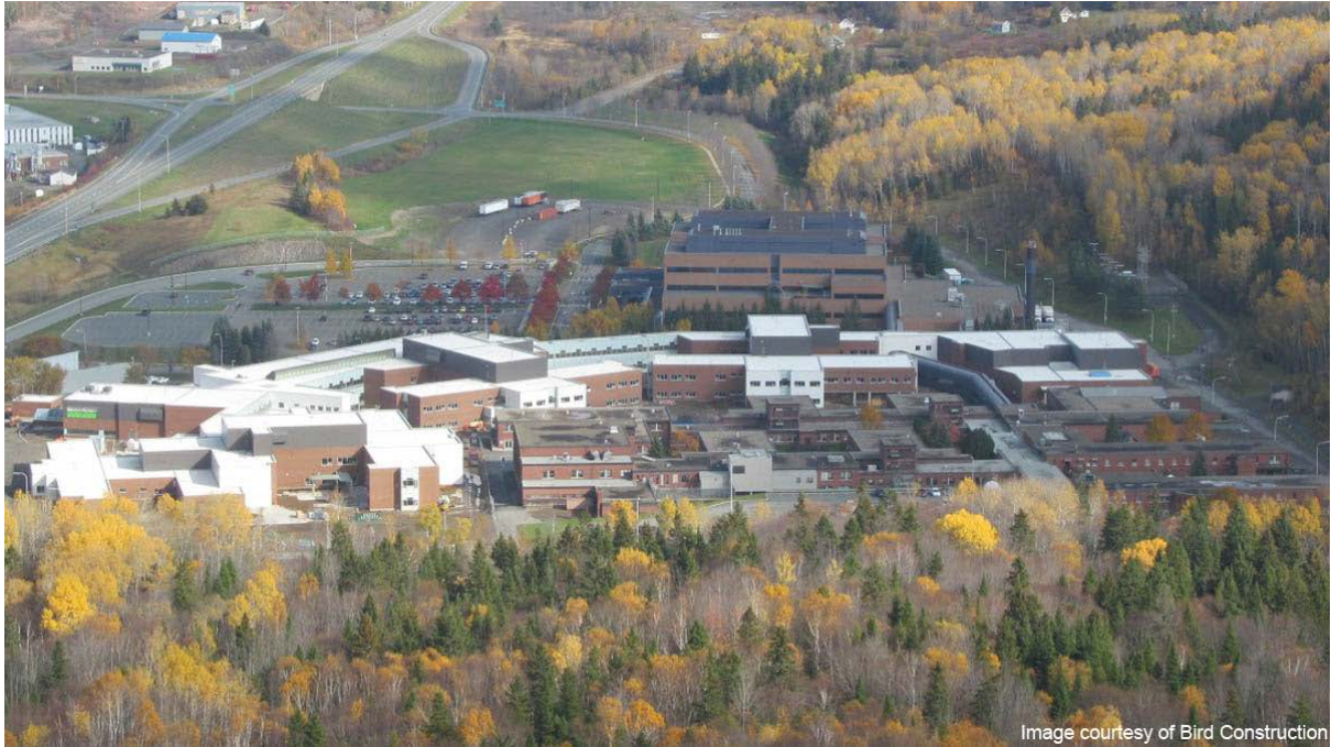
Image courtesy of Bird Construction
