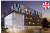
Barking Dagenham & Havering Clinics (LIFT 1 )
