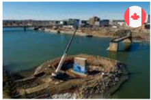
North Commuter Parkway
