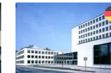
Unna Administrative Centre
