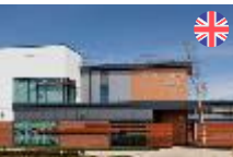
Ayrshire and Arran Hospital
