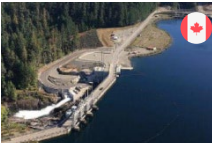
John Hart Generating Station
