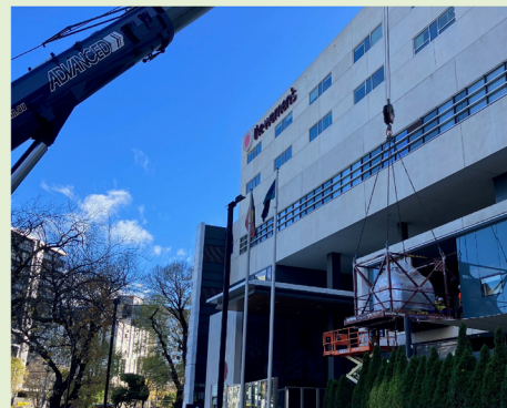
Relocating a MRI machine from Royal Women's Hospital in Australia to India
